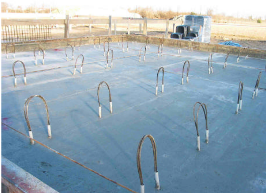
Fig. D.2 Concrete casting with steel lifting rope
