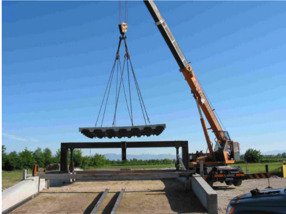
Fig. D.9: Lifting of concrete tests
