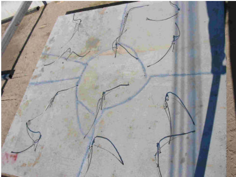
Fig. D.13 Crack line detail on the concrete test n°1
