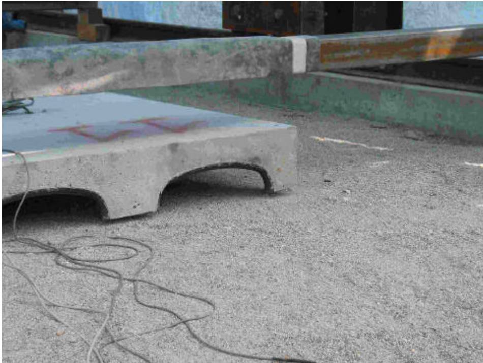
Fig. D.23 Details of lifting the column of the concrete test n°11
