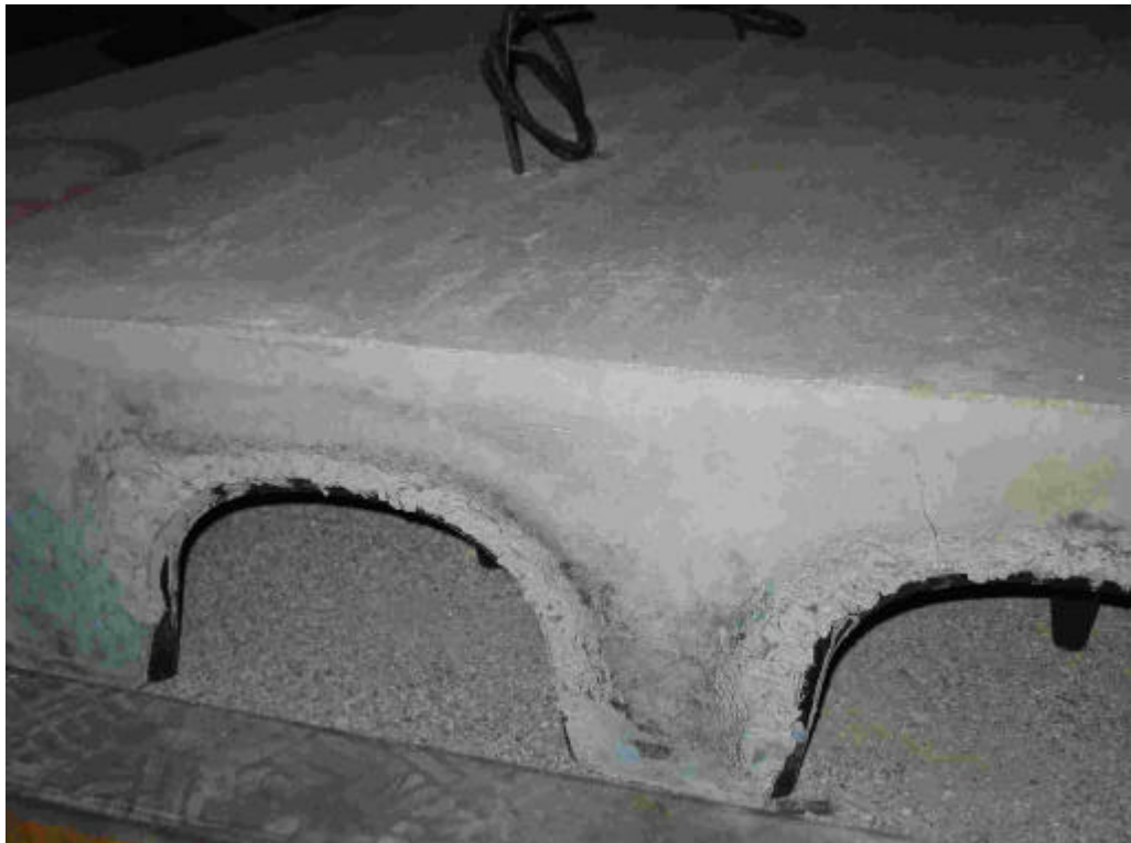
Fig. D.26 Crack line detail on the concrete test n°12
