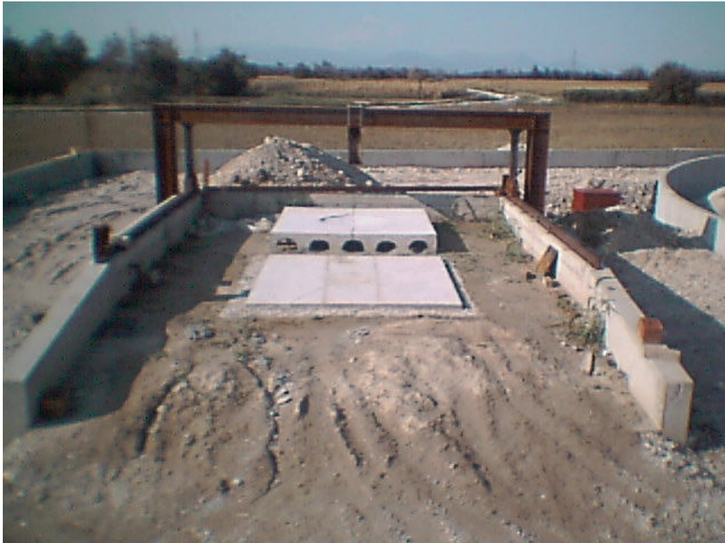
Fig. D.27 Layout tests Cupolex-slab
